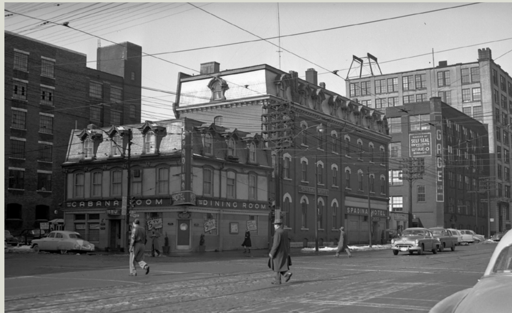
Richardson House (later Spadina Hotel built 1873) | 460 King St W
